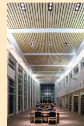
The heart of the new space features a long fluorescent cove that uplights a wood ceiling.
