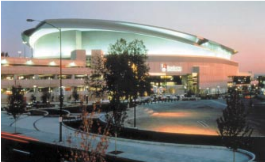
At the Portland, OR, Rose Garden arena, lighting design encompassed the suites, concourses, restaurant, and exterior facade, as well as illumination for the events.
